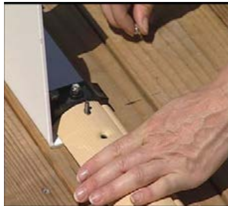
Reinstall the top half of the track guide and tighten down with the 3/8" nylox nut.
