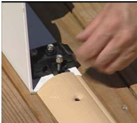
Remove the top of the track guide
