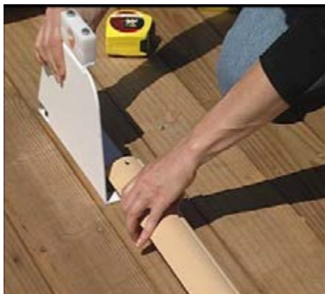
Push the track down over the stud.
