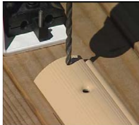
Drill a 1/4" hole into the track.
